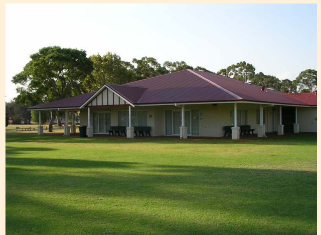
Higgins Park Reserve Club Rooms Building viewed from the southwest. Shows open veranda to three elevations (east, south and west), new gable end facing south and Colorbond clad roofing which replaces the tiled roof which previously facilitated illegal entry to the building.
