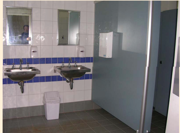
New female toilets showing low maintenance high durability finishes.
